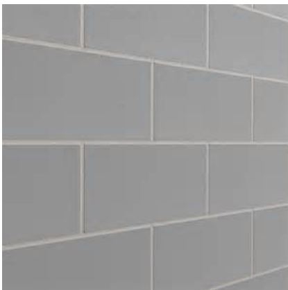
(smooth cmu walls)
